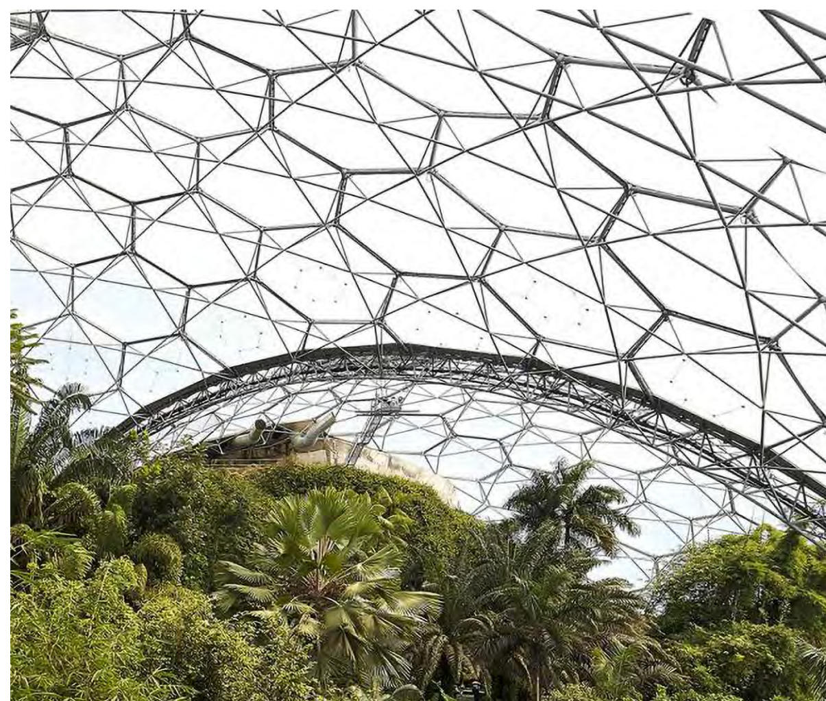
Figura 2: The Eden Project - interno www.arup.com
